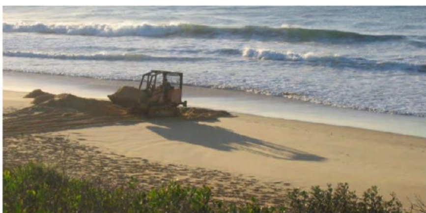
Figure 3-1 Beach Re-profilling using Mechanical Equipment (Carley et al., 2010)
