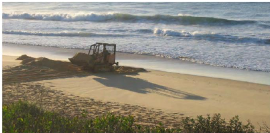
Figure 3-1 Beach Re-profiling using Mechanical Equipment (Carley et al., 2010)
