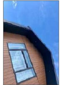
INWOOD ARTIFICIAL TIMBER CLADDING OR ALTERNATIVE
