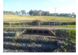
D/S Boundary Road culverts 2 x 1350dia (photograph shows upstream end of culverts);
