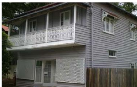
● First floor projection ● Operable windows maximise natural ventilation and prevailing bay breezes ● Chamfer board wall cladding
