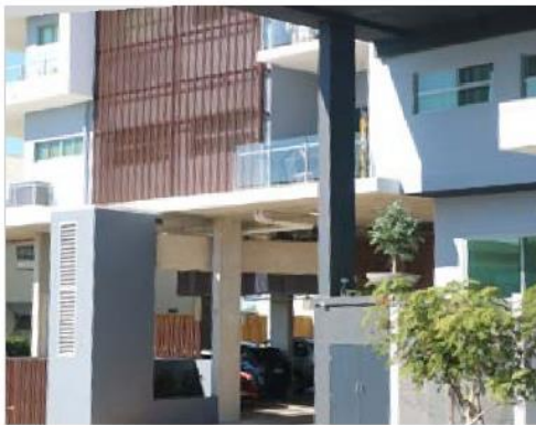
Plant and services screened but still allows for easy access for maintenance and inspection. Services screened to blend in with overall design and simple palette of colours of building.
