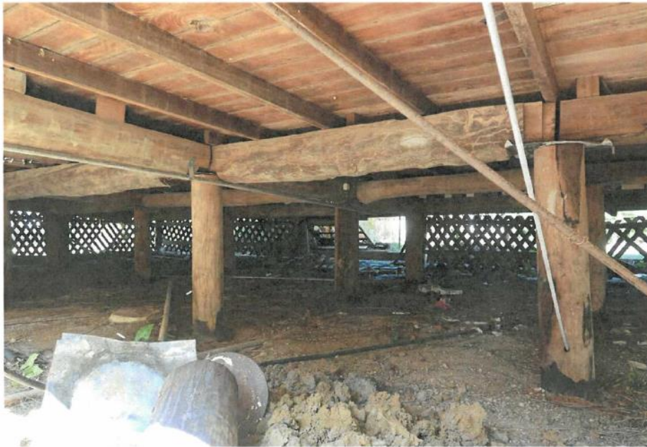
Figure 5: Residence (Main House) sub-floor framing, using early carpentry techniques (Queensland Government, 2021)
