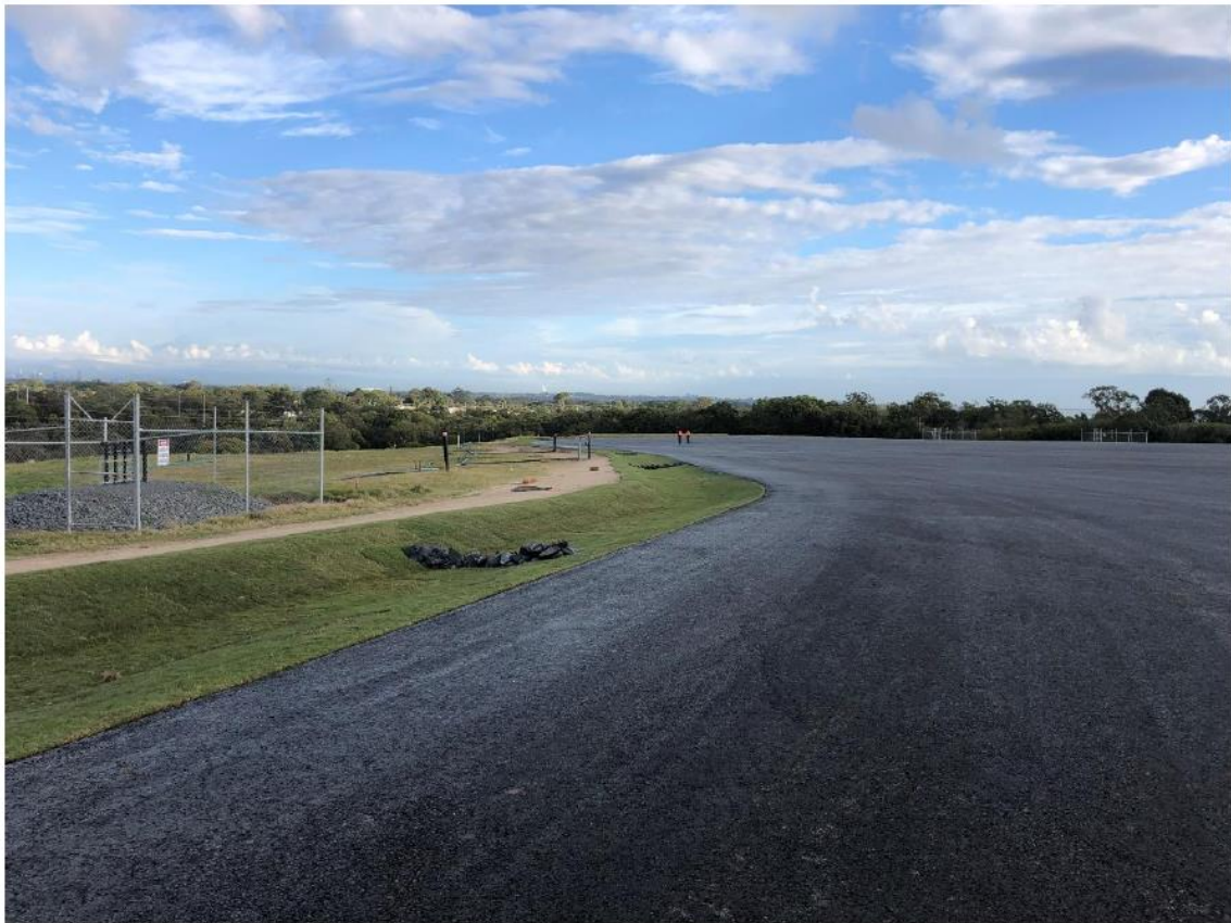
Figure 12: Upgrade of Birkdale Recycling and Waste Centre hardstand using 550 recycled passenger tyres
