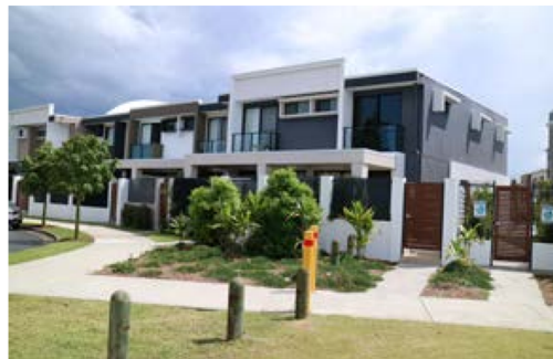
Front doors addressing the street.
