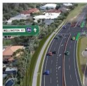
Wellington Street / Panorama Drive road upgrade program
