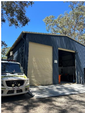
1. Outside of premises.
