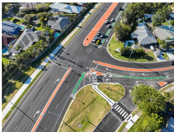
Figure 29: Wellington Street / Panorama Drive upgrades by Council delivered upgrades paths, cycle lanes and crossings
